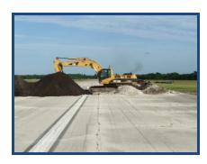
Heavy equipment working on replacing the drainage structures under Runway 11L-29R as part of the Runway rehab project.
