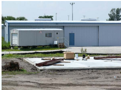
Foundation for new T-hangars
